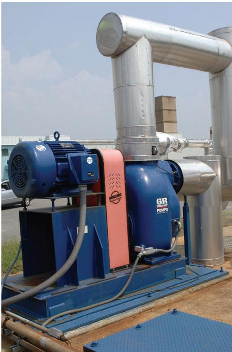
With traditional vertical-line sump pump designs, the pumps remain housed in tight, confined spaces. Therefore, when a team member needed to enter the area for maintenance, a series of confined space entry procedures had to be followed to secure personnel safety. Otherwise, an overhead crane was required to remove the pump from the area, which was a lengthy process – often an all-day procedure.
