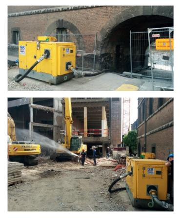
The demolishing site was just next to the River "La Sambre", which was convenient as the pumpset could pump water directly from the river to spray water on the site.
