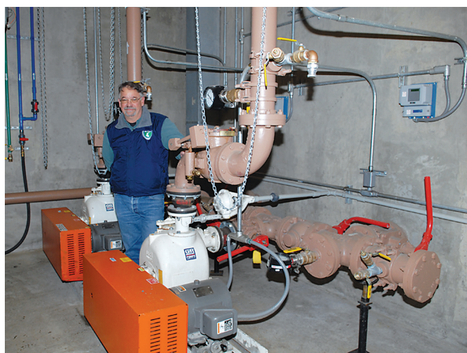
Mike Wageck, District Manager of WPWSD, with the pumps that handle the fluctuating sewage flow from Winter Park, CO.
