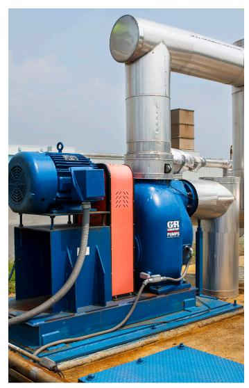
Gorman-Rupp Super T Series® pumps (this an 8" model) were installed for a variety of industrial wastewater applications throughout the power plant.
