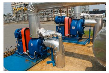
6" and 8" Super T Series pumps work in tandem and are offered in a variety of materials for heavy-duty corrosive and abrasive liquids.
