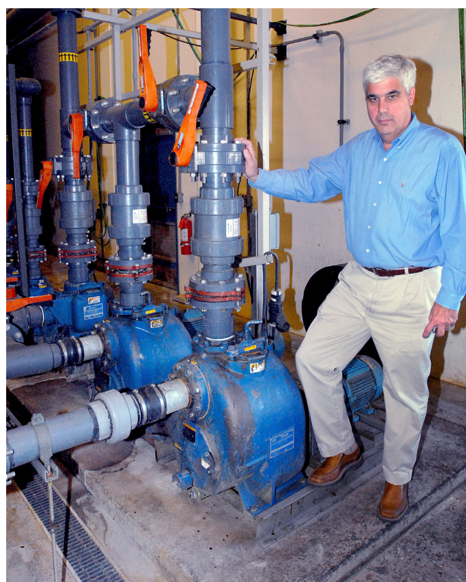
Dave Muskopf stands with one of the five solids-handling, self-priming centrifugal pumps that makes up Ken's Foods' wastewater treatment system.
