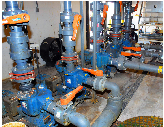
Three 10 Series® and two Super T Series® trash pumps were incorporated into the system for heavy-duty solids-handling capability.
