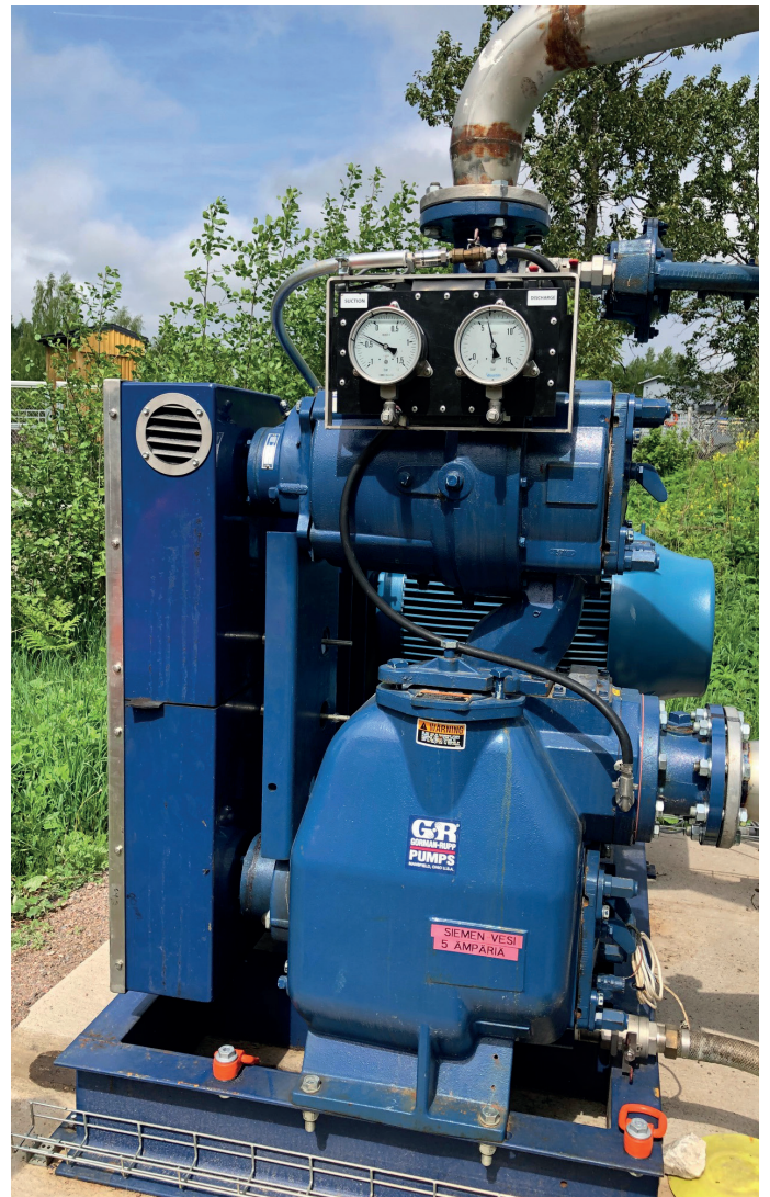
Gorman Rupp VS3A60 self priming centrifugal pump
