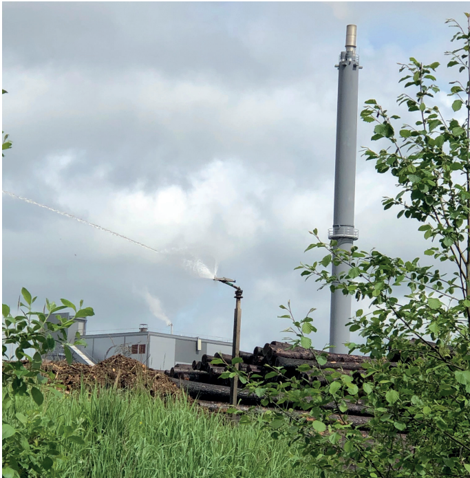
This picture shows the spray beam, keeping the tree trunks wet and being pressure fed by the Gorman-Rupp pump.
