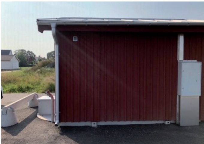
Purpose built enclosure
