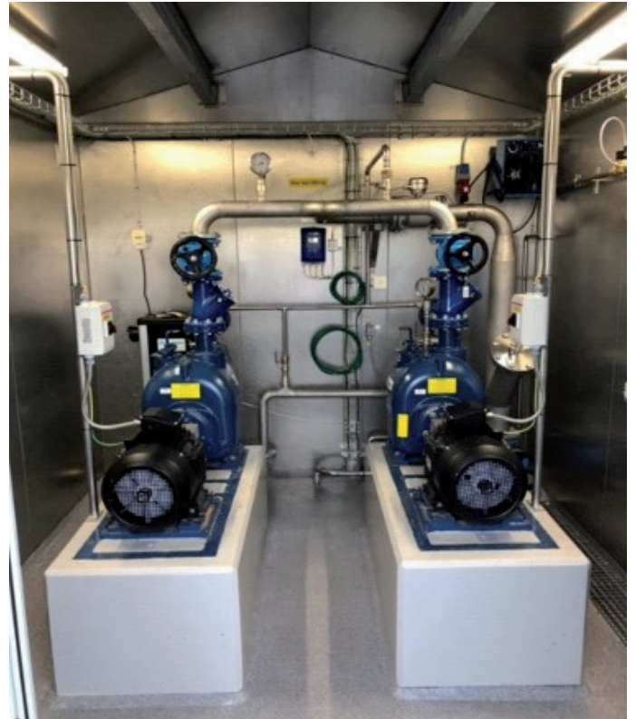
Inside the pump station: two Gorman-Rupp T3C60S pumps in parallel
