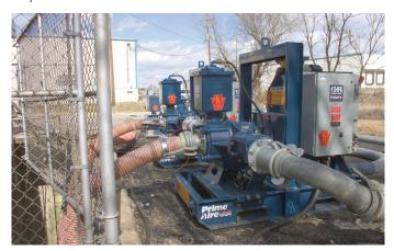
Easy access to electric allowed for three motordriven priming-assisted pumps to be installed for bypass operation during the upgrade. This eliminated the need for refueling engine-driven pumps and reduced noise pollution.
