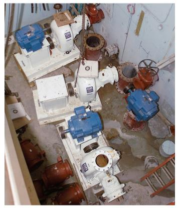
Three 10" Gorman-Rupp Super T Series® pumps being assembled to replace the old dry pit submersible pumps.
