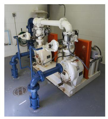
One of the 24 lift stations equipped with a selfcleaning wear plate, this base-mounted station has seen clogging drastically reduced.
