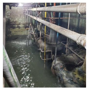
During heavy rain events, incoming flow would overwhelm the outdated pumping equipment often resulting in station flooding.
