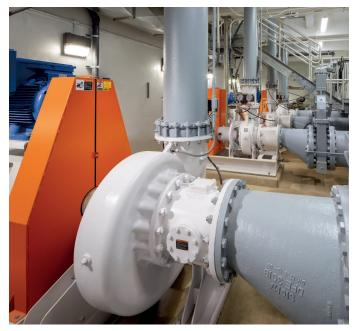
The new installation with two 16" 6500 Series® and two 12" 10 Series® pumps resulted in a much safer and cleaner environment for performing routine pump maintenance and monitoring.
