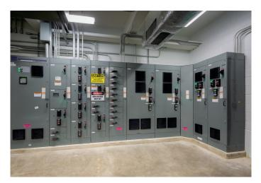
Due to space and structural restrictions, the corner design of the motor control center was crucial in fitting such complex technology into a confined space.
