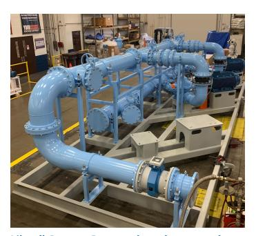
Like all Gorman-Rupp packaged systems, the Southeastern booster station was designed and tested in the Engineered Systems state-of-theart manufacturing facility prior to shipment.
