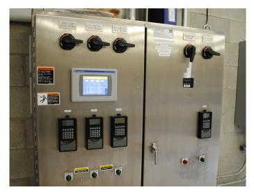
Customized control panel included variable frequency drives (VFD's), PLC with operator interface and operation off suction/discharge pressure transducers.
