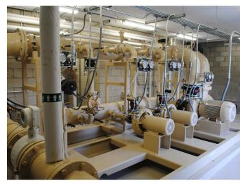
Pressure booster station pump configuration included: (1) Jockey Pump, (2) Duty Pumps, and (1) High Flow Pump to accommodate long-term water usage over 60 PSI.
