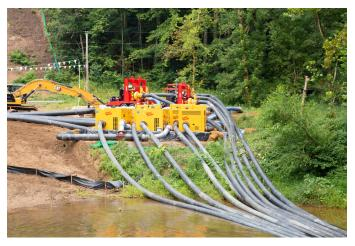
The quality built into Gorman-Rupp rental pumps makes them ideal for sewage and river bypass projects. This setup is bypassing a large creek during the installation of an underground power line.
