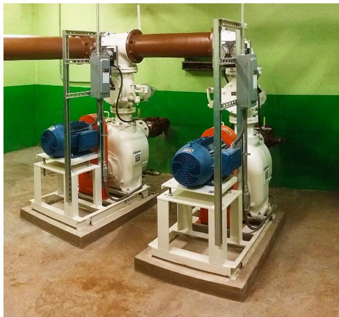
**Gorman-Rupp Super T Series® pumps can be mounted above the liquid being pumped. Should service or maintenance be required, it can be easily performed using common hand tools and without disconnecting piping.**
