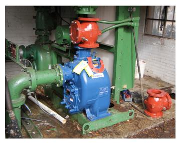
Old versus new. One of the old pumps from the original station was still pumping reliably after forty years of service. The entire station was completely retrofitted in just under five hours.
