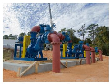
In 2013, the City of Fairhope began construction upgrades to their wastewater treatment plant. Based on their success with T Series® and Super T Series® products, a majority of pumps installed throughout the facility were Gorman-Rupp self-priming centrifugals, including these four 12" 10 Series nitrate recycle pumps.
